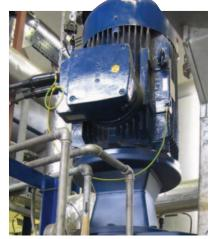
and electric motor technology, which saves energy by using a smaller 15kW motor.
